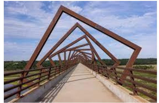
Figure 6.4 – High Trestle Bridge Source: Boone County
